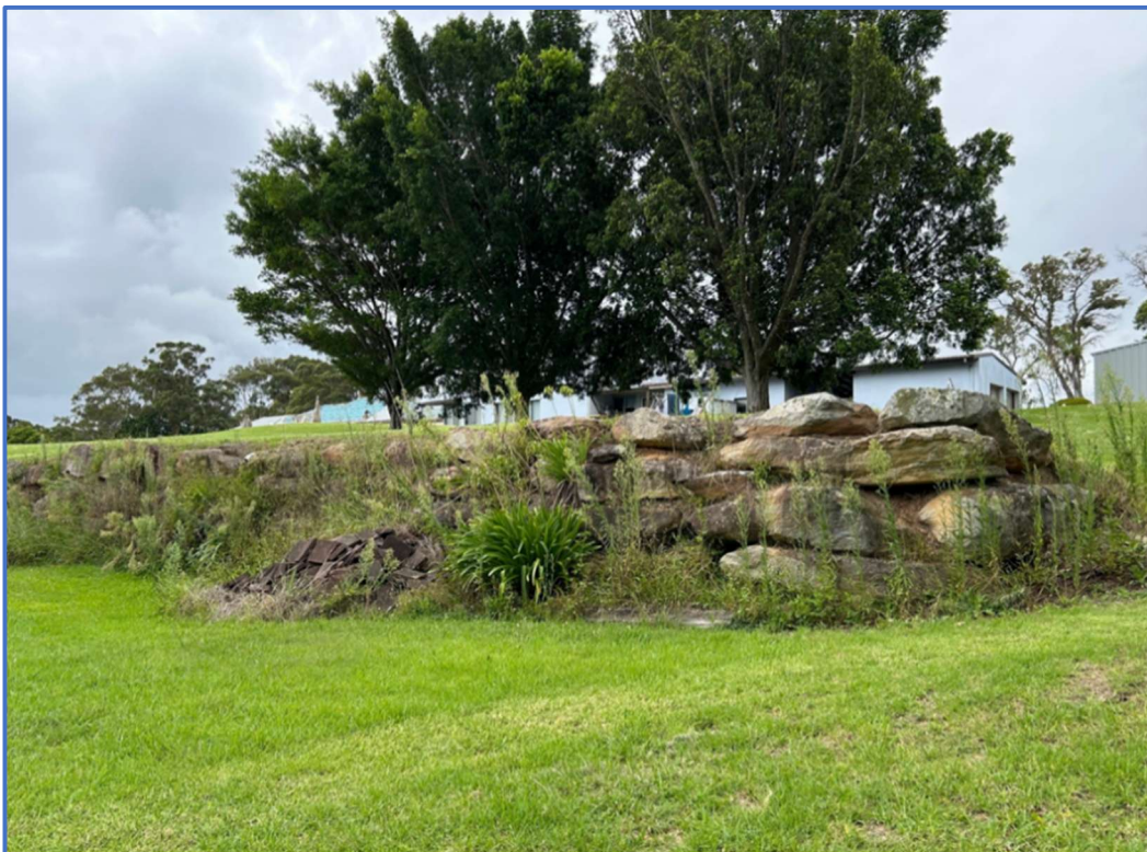
Figure 7 – Exiting landform terracing supported by a 2 m high boulder wall at No. 614 Old Northern Rd
